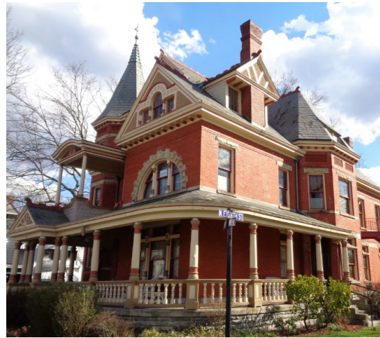
On this Gothic/Gothic Revival, while it is a brick structure, note the use of earth tones for body, trim and accent. Red brick for the body, complimented by browns and beiges as trim, and then returning with muted pale reds for accents to compliment the brick body.
